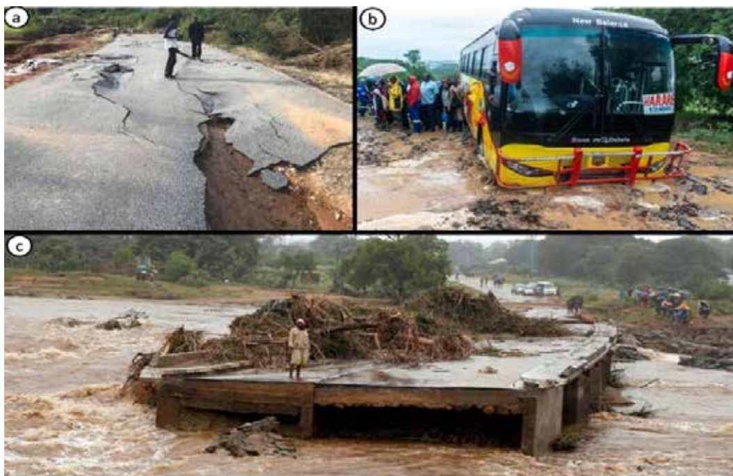
Figure 10. Road destruction from cyclone Idai (2019) in Eastern Zimbabwe: (a) road damaged (b) softened road surface causing busses to sink (c) Bridge washed away.
