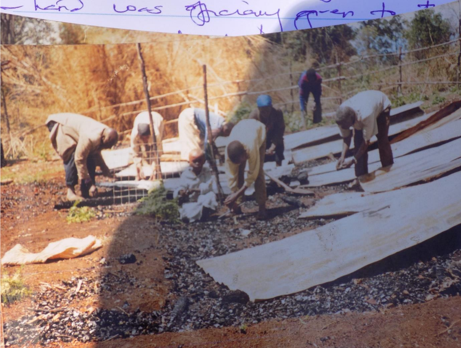
Parents collecting remains of construction materials after school demolition
