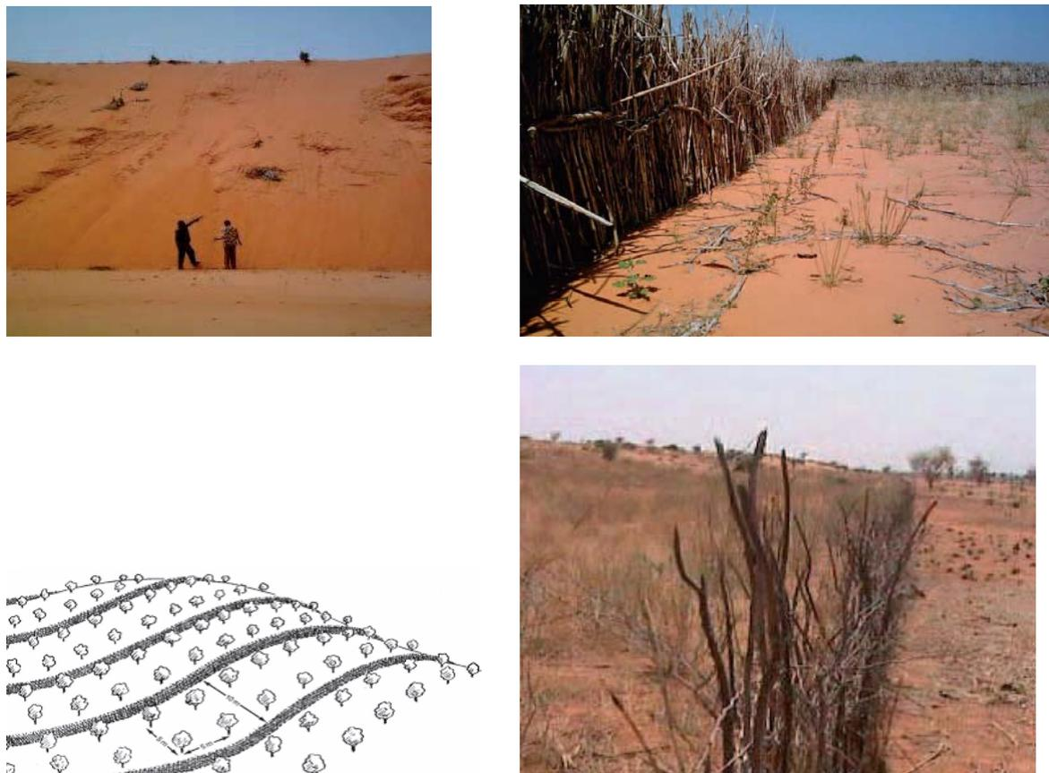
**Figure 9. Dune stabilisation using hedges and palisades, Niger (wocat/fao, 2011)**
