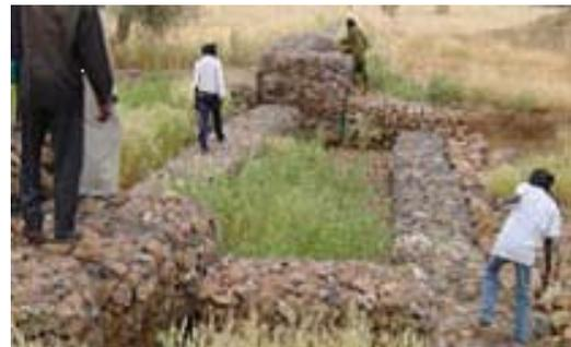
**Figure 7. Construction of permeable rock dams**
