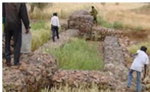
Figure 7. Construction of permeable rock dams
