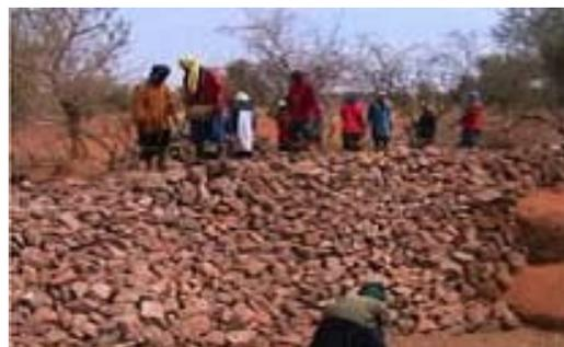
Closing off a gully with a permeable rock dam (PGRNG, Mauritania).
